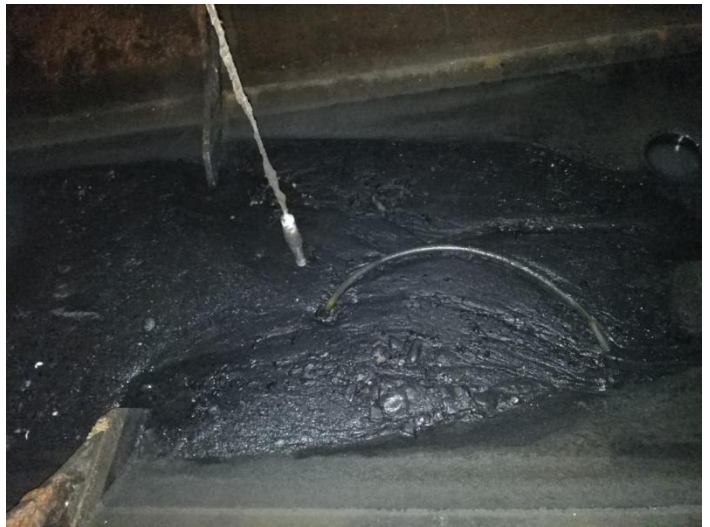
Sludge was really tick , able to damage discharge pump vanes and clog one way valve diaphragm Sensor head was dirty
