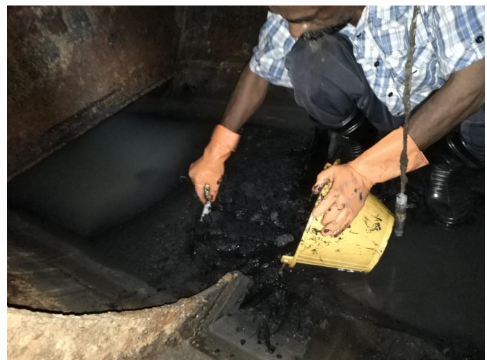
Sludge was really tick , able to damage discharge pump vanes and clog one way valve diaphragm Sensor head was dirty
