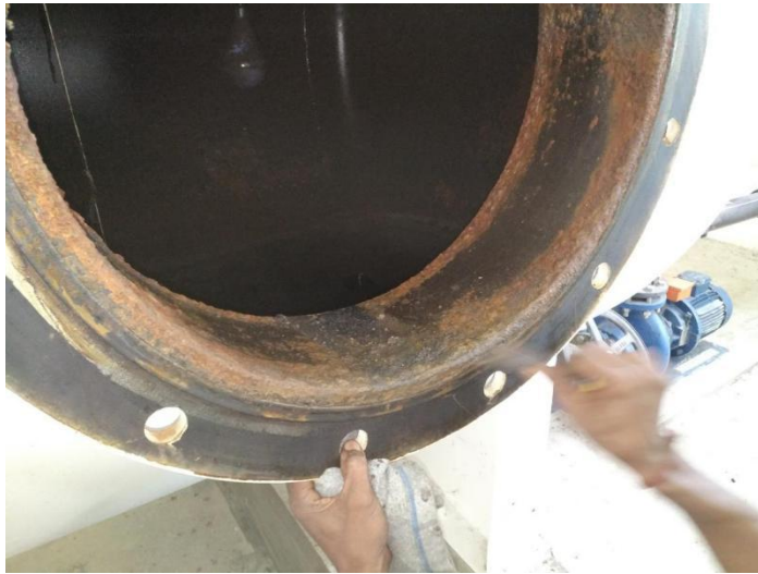
All bolts and nuts tightness tested
