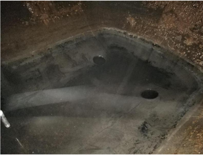
Sensor head washed clean , Flushing work done
