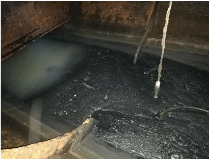
Sludge was really tick , able to damage discharge pump vanes and clog one way valve diaphragm Sensor head was dirty
