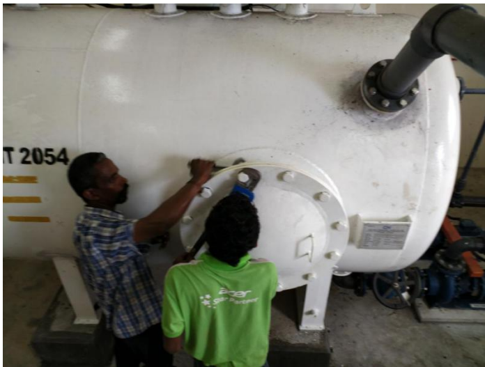
High vacuum pressure leak test carried out
