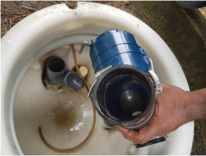
Very low on suction – valve opened and checked for blockage
