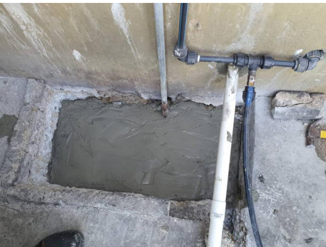
Grease Trap base concreting works
