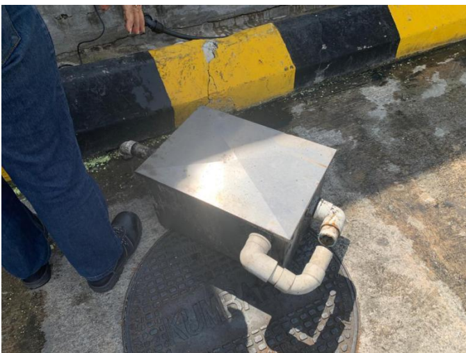
Damaged Grease Trap removed
