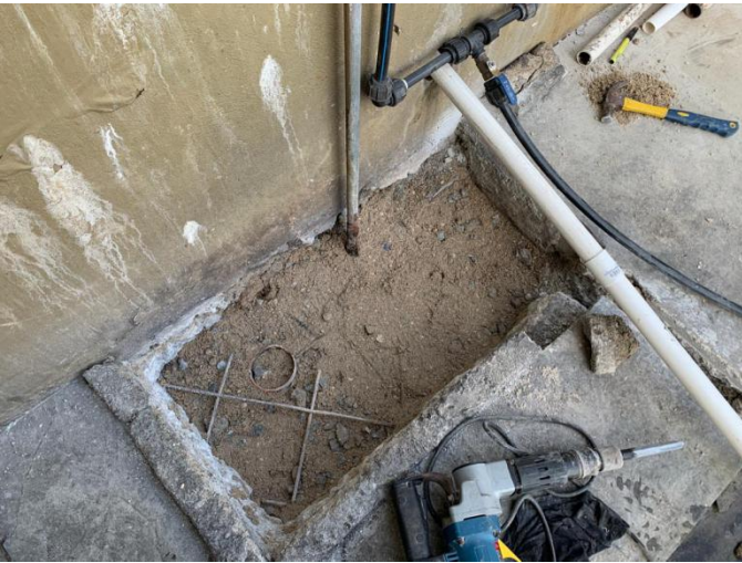
Grease Trap base Hacking works
