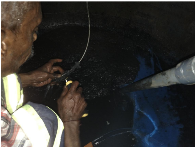
Sensor was tied up with a bundle of strings , carefully removed
