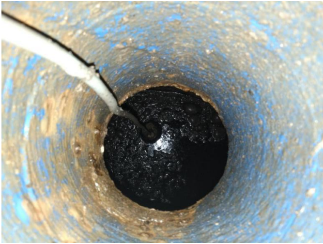
View from sensor manhole
