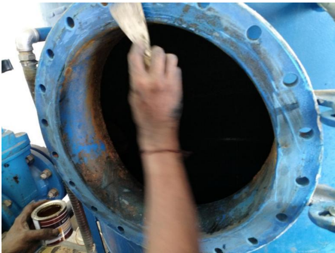
Gasket adhesive applied
