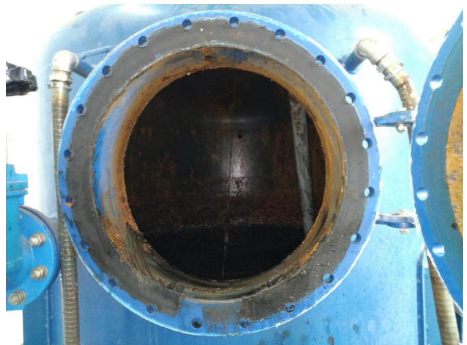
We began opening the manhole on the vacuum vessel , gasket was damaged ( need replacing )
