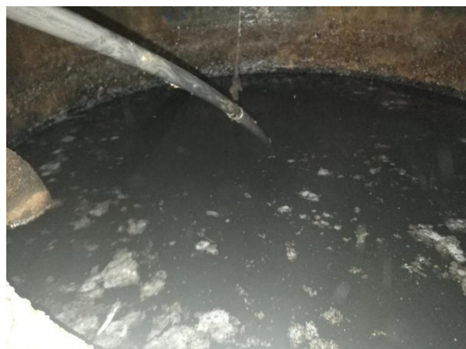
Sewage water manually removed and removed 1 feet height of sand collected at bottom portion of the vessel
