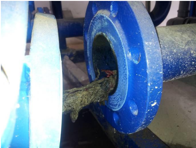
A few batches of strings n cloths found in the discharge line
