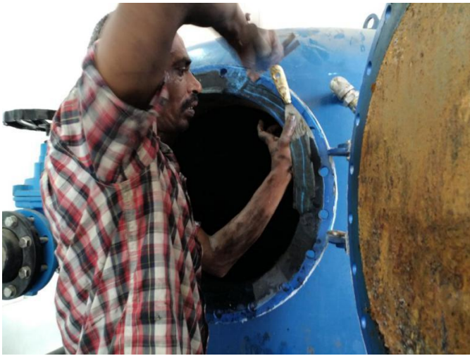
Old gasket removed and surface sanded
