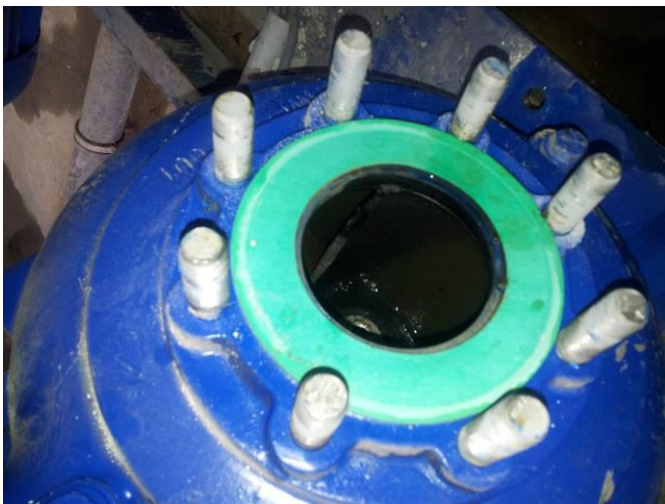
Discharge pump does not show any sign of damages or stuck
