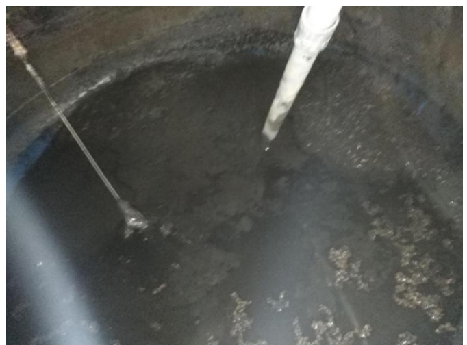
Sewage water manually removed and removed 1 feet height of sand collected at bottom portion of the vessel
