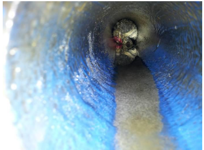
Compacted batches of strings n cloths
