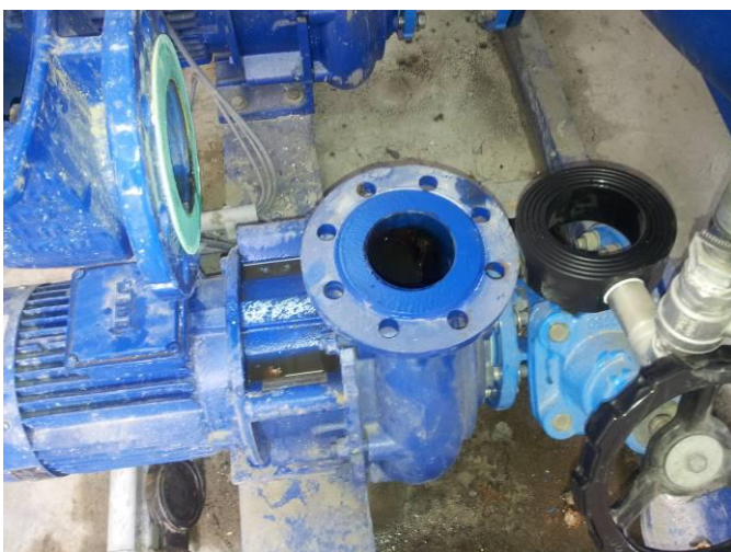
Discharge pump looks clean and no sand detected
