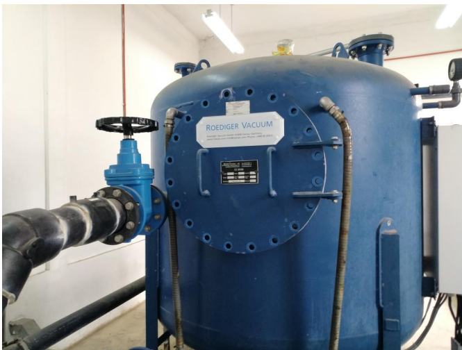
We began opening the manhole on the vacuum vessel , gasket was damaged ( need replacing )
