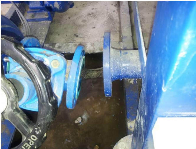
A few batches of strings n cloths found in the discharge line
