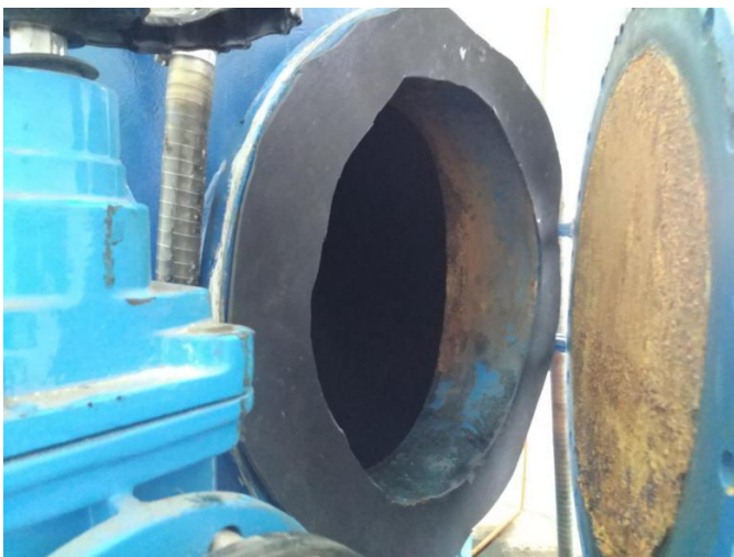
Customized larger and thicker rubber gasket used
