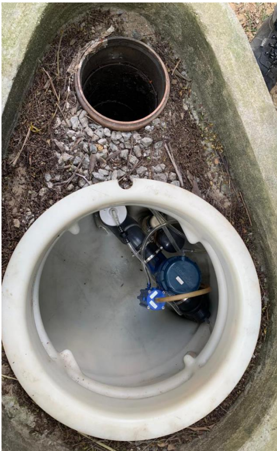
Chamber pod self-evacuation unit properly installed , this will eliminate any water ponding in pod due to heavy rain
