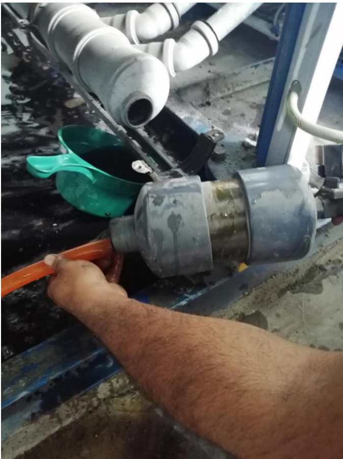
Compacted debris removed from the condensate trap
