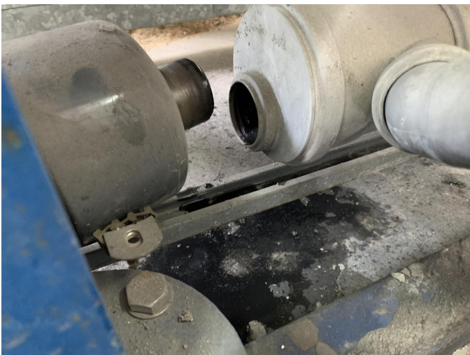
We removed the condensate trap to inspect further
