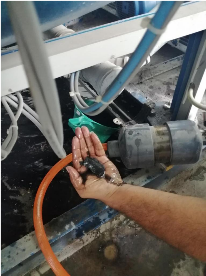
Compacted debris removed from the condensate trap
